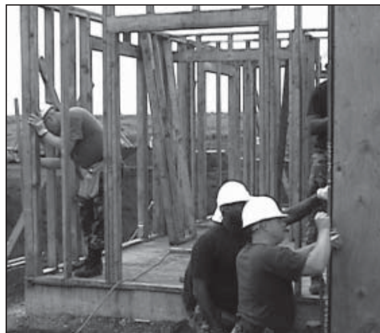
From left, Master Sgt. Daryl Waters, Senior Airman Christopher Powell, Tech. Sgt. Eric Loper and others work on squaring exterior framed walls on a housing unit.
