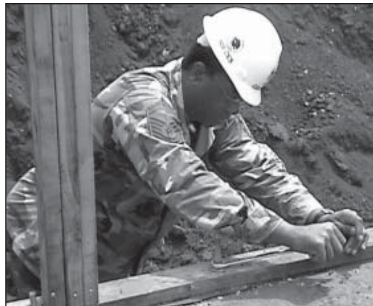
Senior Master Sgt. J. C. Collins tightens anchor bolts to secure the exterior walls of a housing unit to the concrete floor.
