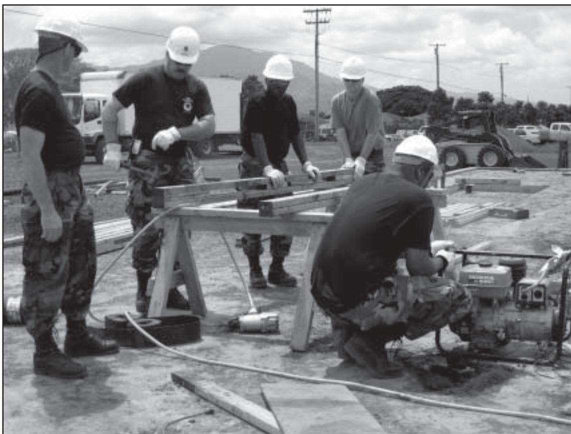
From left, Tech. Sgt. David Barber, Senior Master Sgt. Don Fenn, Senior Airman Allan Jordan and Staff Sgt. Don Fykes construct framing components for the walls of a housing unit while Master Sgt. William James, kneeling, adjusts the generator being used to supply power for tools at the site.
