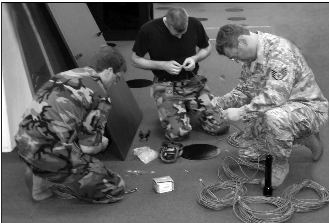
Above, Staff Sgts. Jeff Pierce (left) and Keith Rudolph (right), assisted by a Ramstein AB Airman, create cables for the project rewiring and converting five racks of network servers to four.
